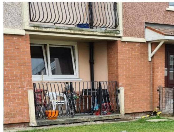
Balcony with combustible items and gas barbecue
