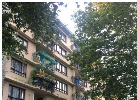
Balcony with overhanging combustible items stored
