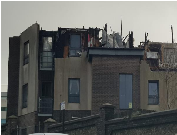
Damage following balcony fire in Brighton September 2019
