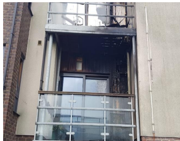
Timber clad balcony – close-up evidence of the fire spread
